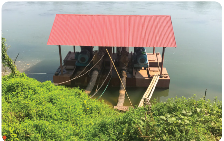
Support for replacement of diesel pumps with electric pumps in Lao PDR, leading to cost savings for farmers and environmental benefits
