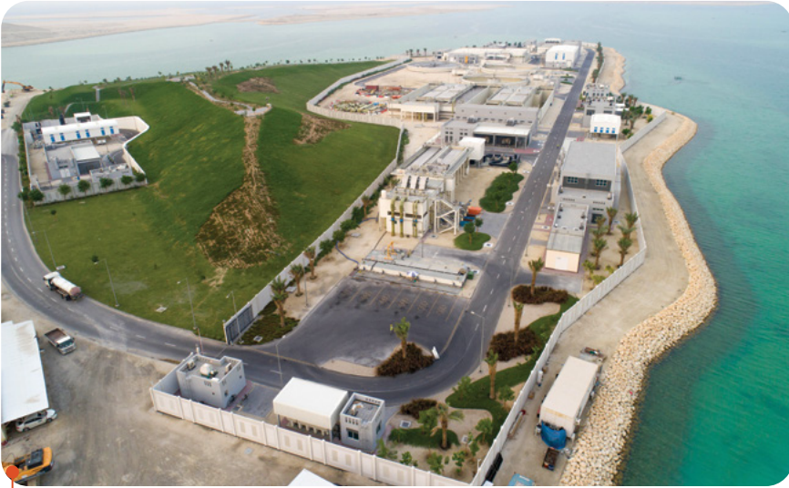
Assisted an Indian company to execute critical wastewater treatment infrastructure for a major urban development project in Bahrain
