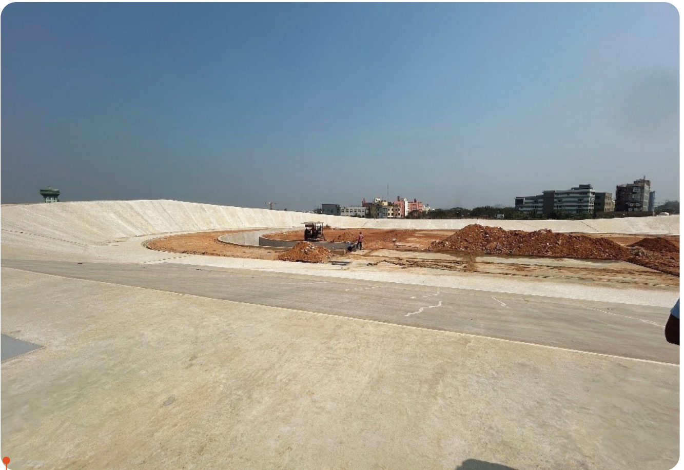
Construction of the cycling velodrome underway in Bhubaneswar, Odisha
