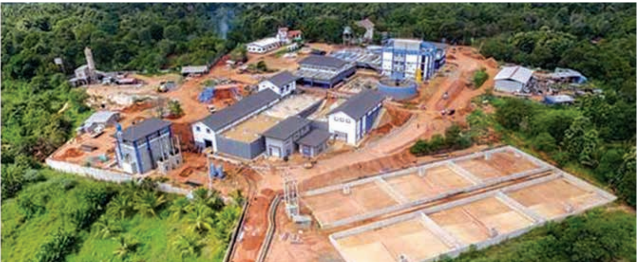
A project for a 30 MLD water treatment plant and distribution to 9 reservoirs across Dambulla region in Central Sri Lanka being executed by VA Tech Wabag Ltd., is financed under the Bank's Buyer's Credit Programme.
