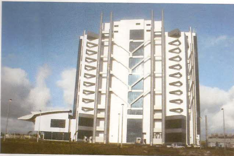
Eleven-storeyed Ebene Cyber City Tower under construction by Larsen & Toubro Ltd. and Shapoorji Pallonji & Company Ltd., in Mauritius. Exim Bank has provided guarantees and bridge finance to the Indian companies for this project, which is being financed under a Government of India loan of US$ 100 mn to Government of Mauritius.
