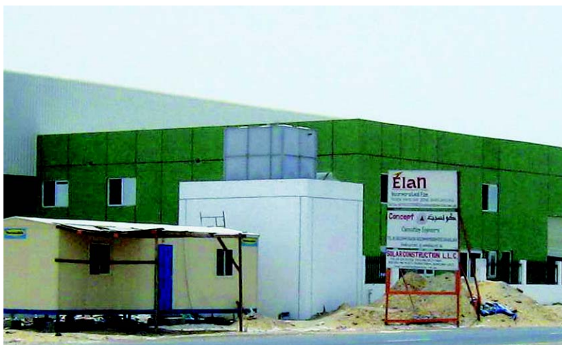
A new production unit being set up in Sharjah by Elan Incorporated, FZE, wholly owned subsidiary of Time Technoplast Ltd., with financial support of Exim Bank for manufacture of liquid packaging (HDPE Drums) and other plastic molded products.
