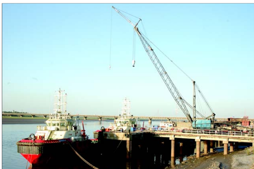
ABG Shipyard Ltd., Surat, is one of India's major private sector shipbuilders, supported by Exim Bank for its export business through long term export credit and guarantee facilities.
